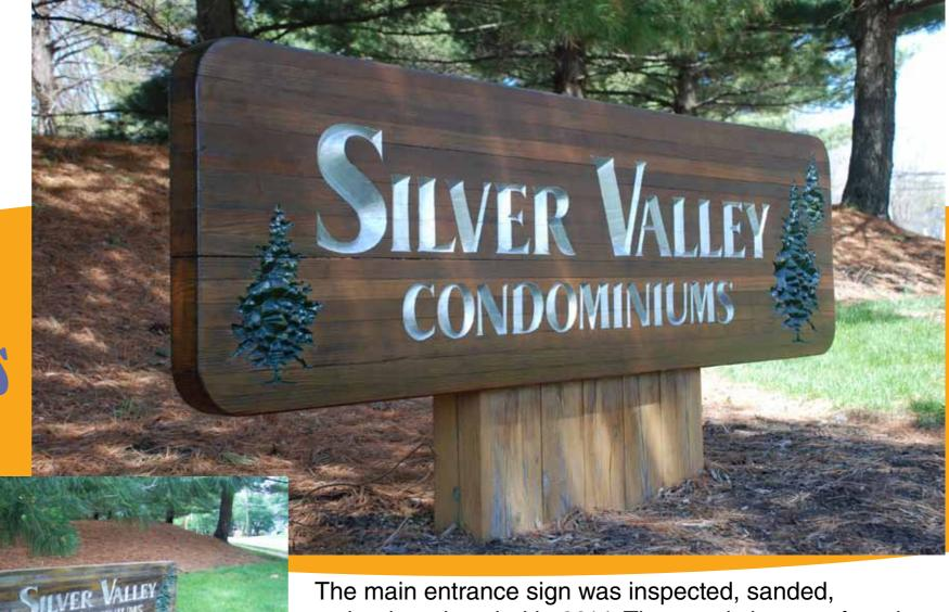
The main entrance sign was inspected, sanded, stained, and sealed in 2014. The wood sign was found to be structurally sound and serviceable for many years, with continued, periodic maintenance. Same for street entrance signs.
