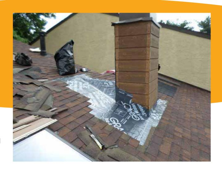
Unlike the original, substandard roofing installation, the new shingles were nailed over felt, and self-sealing ice guard membrane was installed six feet above all gutters, and in other critical areas.
